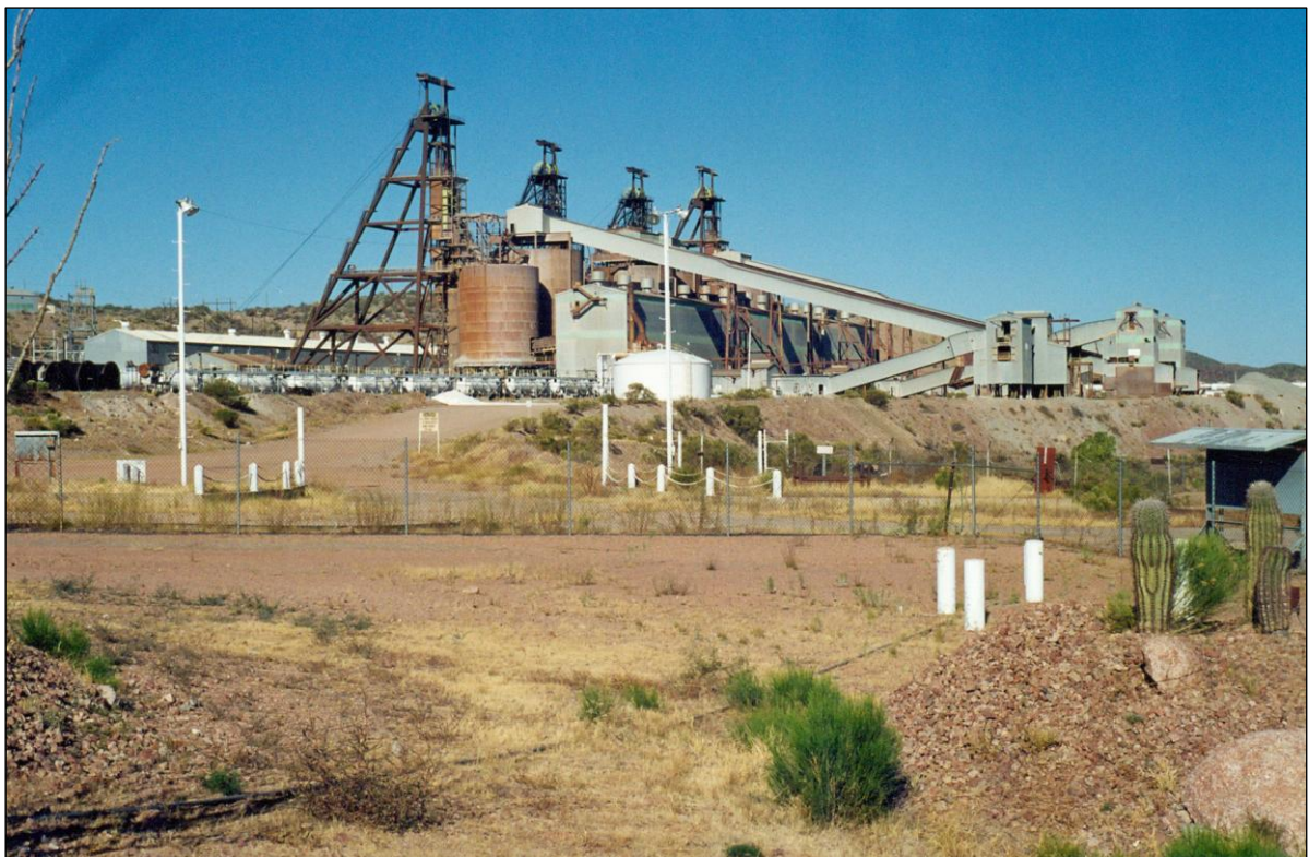
Figure 6-4: Production Shaft Headframes at San Manuel, Showing the Surface Infrastructure Associated with Underground Hoisting Operations
